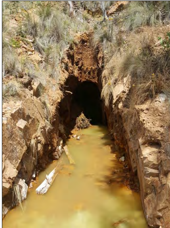
Plate 1. AMD from the main adit at the Nevada mine site, prior to remediation works.
