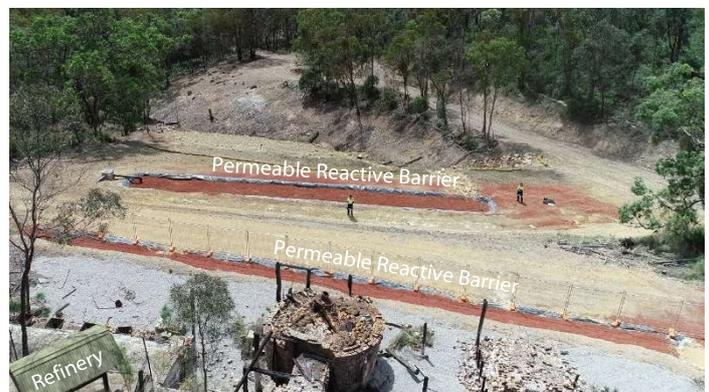
Figure 1. Aerial view of the refinery structures (foreground) and the two lined PRB channels containing reactive substrate (red).
